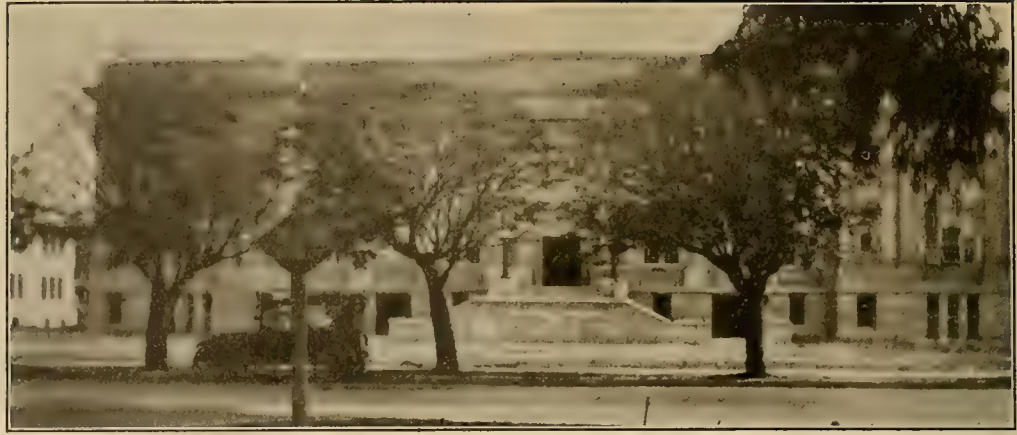
Selma High School, New Science Hall, in Fresno County Free Library.
